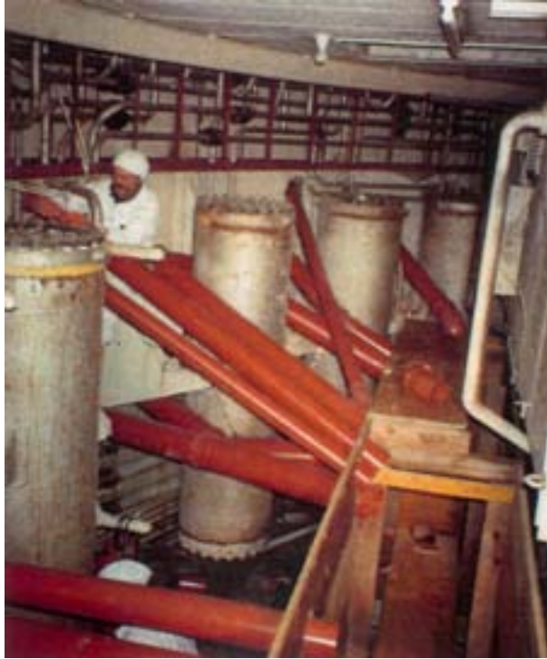
FIG. IV-9. Installation of a new cavern drainage system at Lucens.
