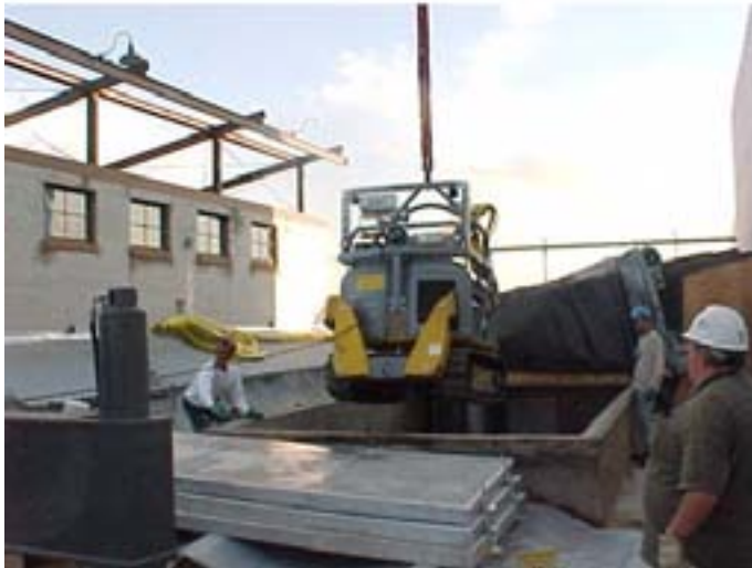
FIG. 14. Lowering of the remotely operated dismantling device (BROKK) into the BGRR duct, Brookhaven, New York, USA.
