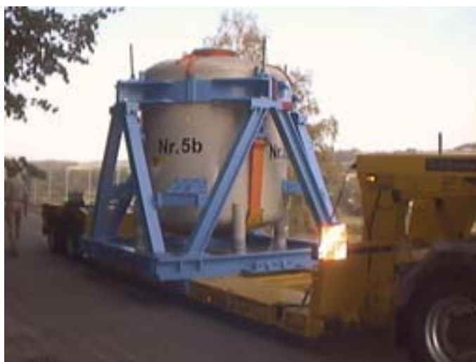
FIG. IV-7. Special containers for transportation of large components from the former research reactor at Lucens to the Swiss central interim storage facility (ZWILAG).
