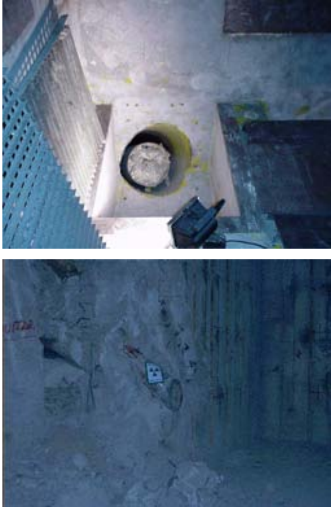
FIG. III-3. The two ends of the embedded pipe at Vandellós 1 nuclear power plant shown in Fig. III-2 (a).
