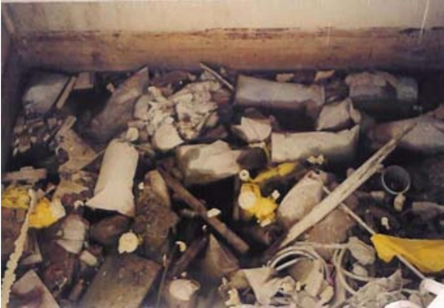
FIG. VII-11. Example of the wastes inside the SRWSF tanks at the A-1 nuclear power plant at Jaslovské Bohunice.
