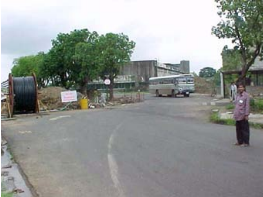
FIG. VIII-2. View of the main road blocked off and traffic diverted to a bypass road in order to allow access to the pipes below the main road at the Cirus reactor, India.
