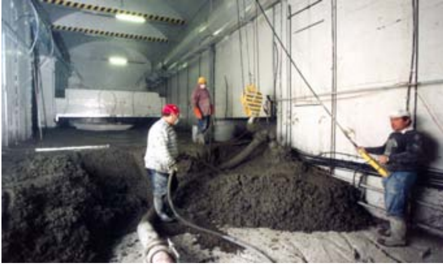
FIG. IV-11. Refilling of caverns with concrete at Lucens.
