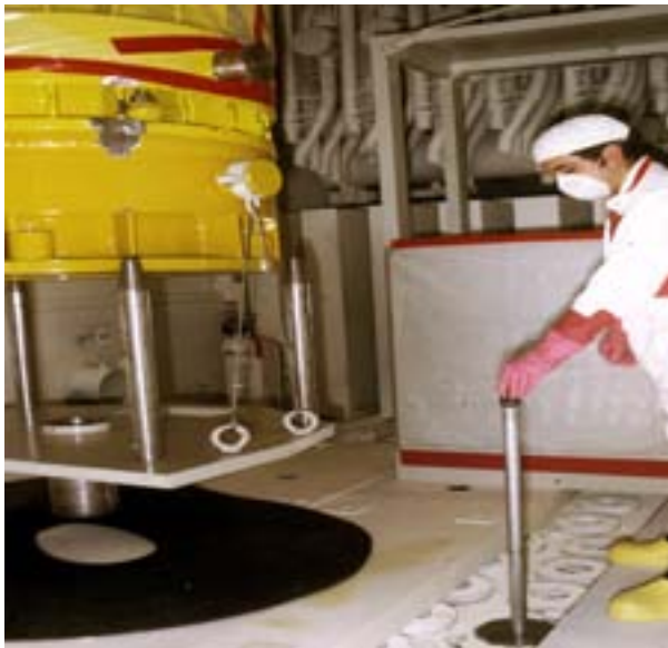
FIG. IV-4. The provisional docking station on top of the core at Lucens.
