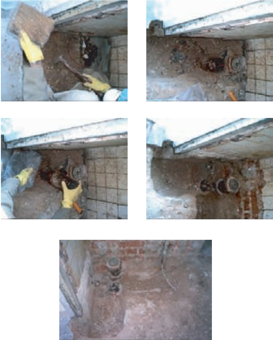
FIG. IX-5. Removal of traps and surrounding material at INOR, Havana.
