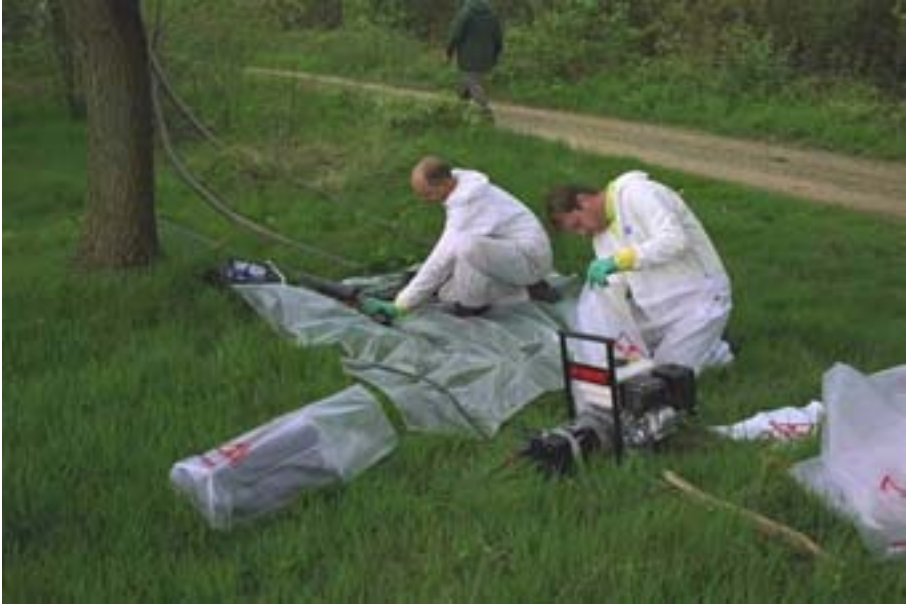
FIG. X-2. The segments are cut on-site and placed in plastic bags, Molse Nete, Belgium.
