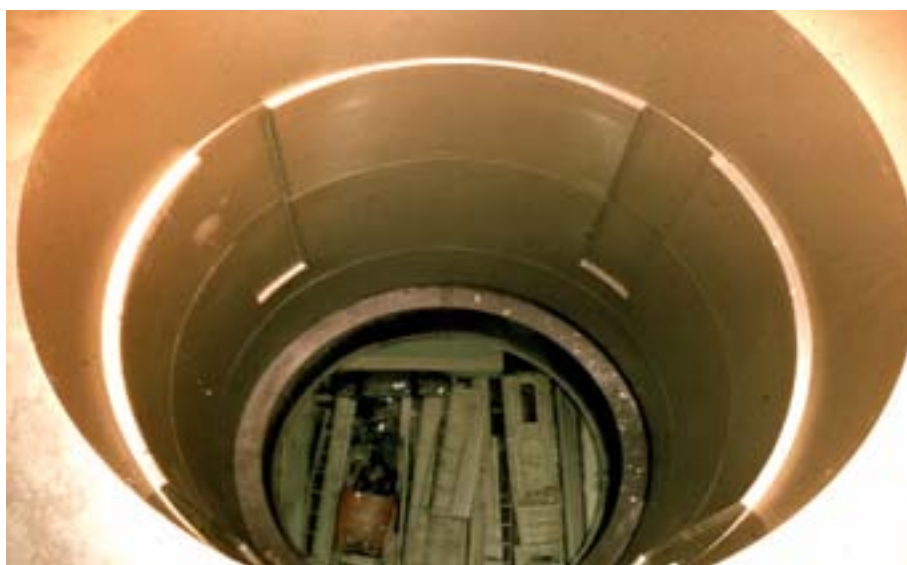
FIG. IV-8. The emptied and cleaned-up reactor pit at Lucens.
