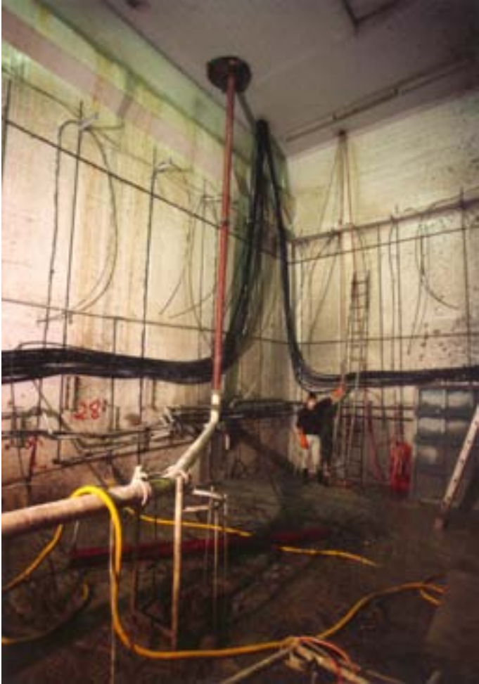
FIG. IV-10. Installation of a grouting hose system at Lucens.
