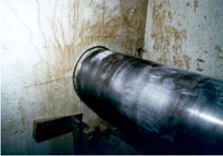
FIG. 13. Segmentation of a steam converter embedded pipe.
