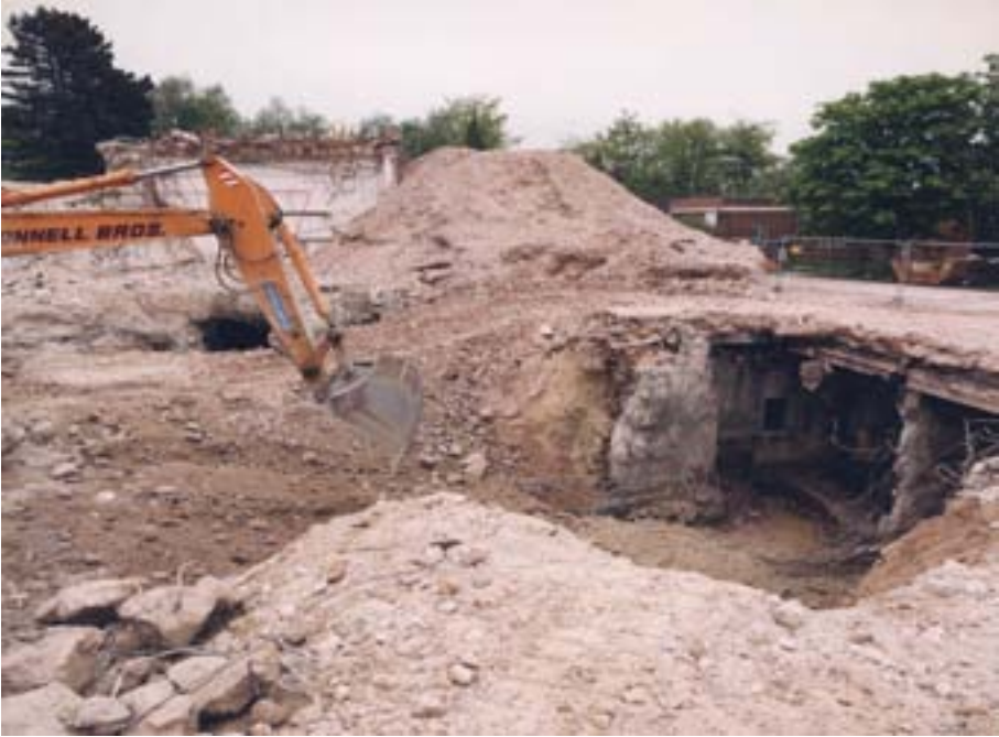
FIG. V-4. Demolition of the BEPO outlet duct at Harwell, UK.
