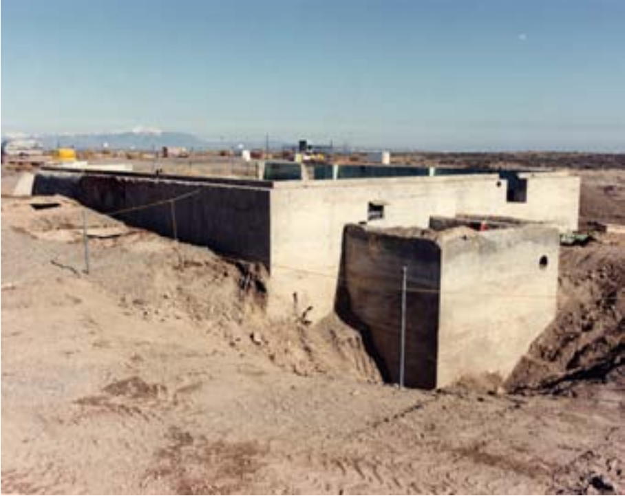
FIG. 5. Removal of contaminated soil around the boiling water reactor (BORAX) turbine building at Idaho National Engineering Laboratory, Illinois, USA.
