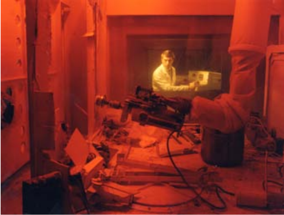
FIG. 25. An ARTISAN manipulator at work during hot cell decommissioning in Building 540, UK. Courtesy: AEA Technology.
