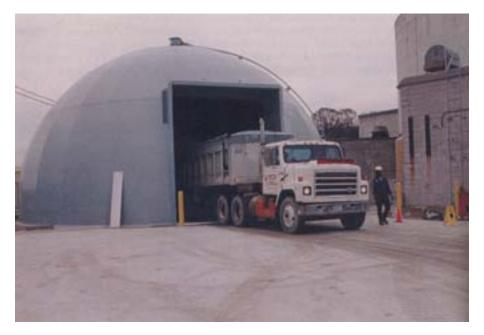
FIG. 5. Vaporsphere, formerly used as an auxiliary facility to the CP-5 reactor, was free released and reused by ANL Operational Services as a storage facility.
