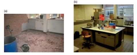
FIG. I.B–6. (a) SCK•CEN metallurgy building, controlled area. Removal of contaminated parts from walls and floor. (b) VITO materials and process technology building, refurbished laboratory.
