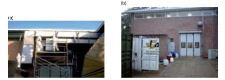
FIG. I.B–2. (a) SCK•CEN metallurgy building, hall-1-bis outside. Removal of contaminated ventilation ducts. (b) VITO materials and process technology building, process hall outside.
