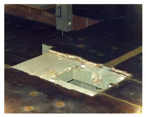
FIG. 14. RB-2 reactor, Montecuccolino, Italy. Reactor hall floor after removal of the reactor (1986).
