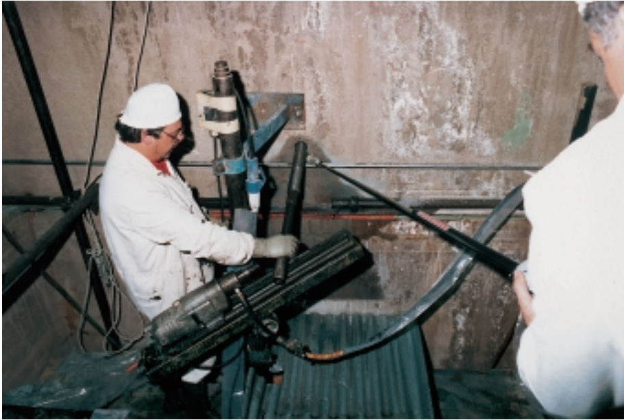
FIG. I-5-1. Garigliano NPP: taking samples from reactor biological shield.
