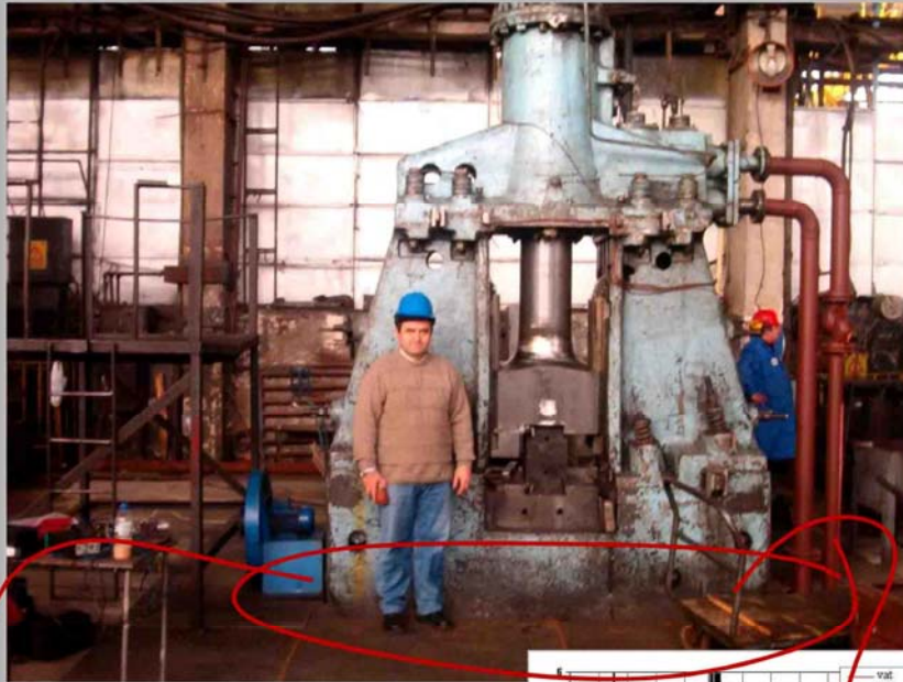
Rehabilitated forging hammer fundation
